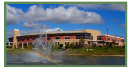
Bay Park Community Hospital
